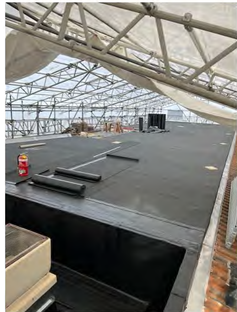
10026 Dunedin Hospital Critical Infrastructure Works Oncology roof replacement
