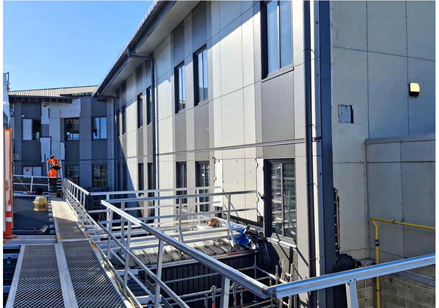
102101 Manukau Elective Surgical Hospital Building Recladding, Manukau Health Park
